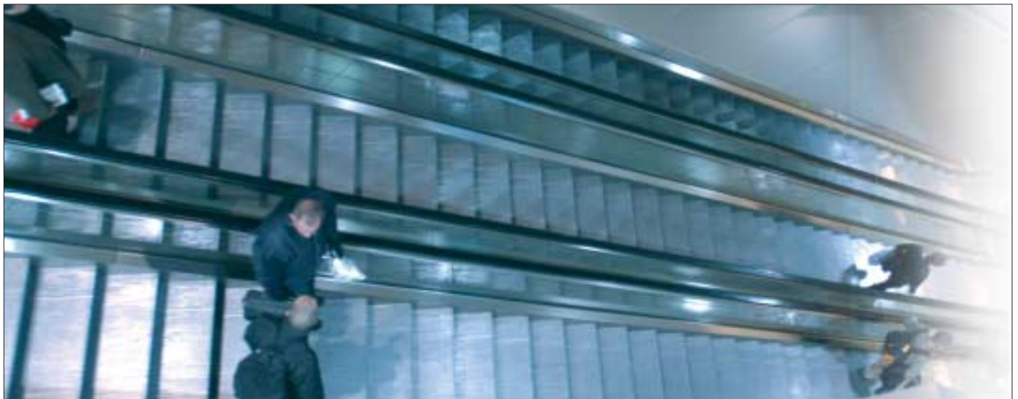
Impressive banks of escalators can be found in public places such as underground stations or airports: Europe on the move
